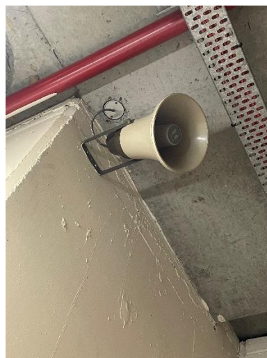
Figure 19: EWIS horn speakers and strobe lights
