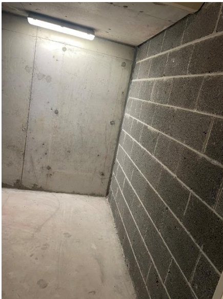
Figure 3: Fire egress stair not containing fire hydrant.
