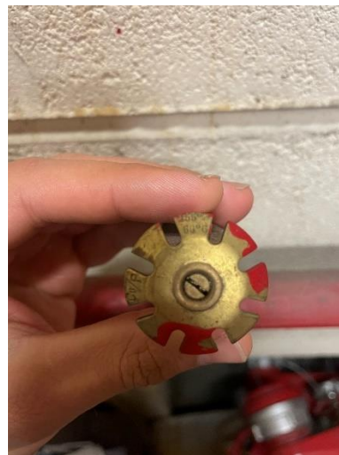
Figure 8: Sprinkler heads example and sprinkler pipes
