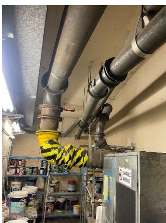
Existing Mild Steel sewer drainage.
